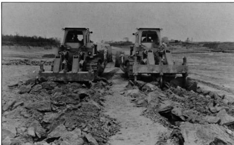
A major problem in land rehabilitation is soil compaction. Mechanical ripping using an agriculture subsoiler (above), deep tillage cultivator or crawler tractor (below) is required to ameliorate adverse soil compaction problems (bottom photograph courtesy of Crothers, Caterpillar Dealers, Concord)
