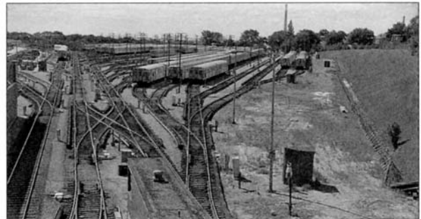
Photograph 5 Site of the Toronto Transit Commission's Greenwood subway yard. The depression offers protection to the subway cars parked and serviced here.
