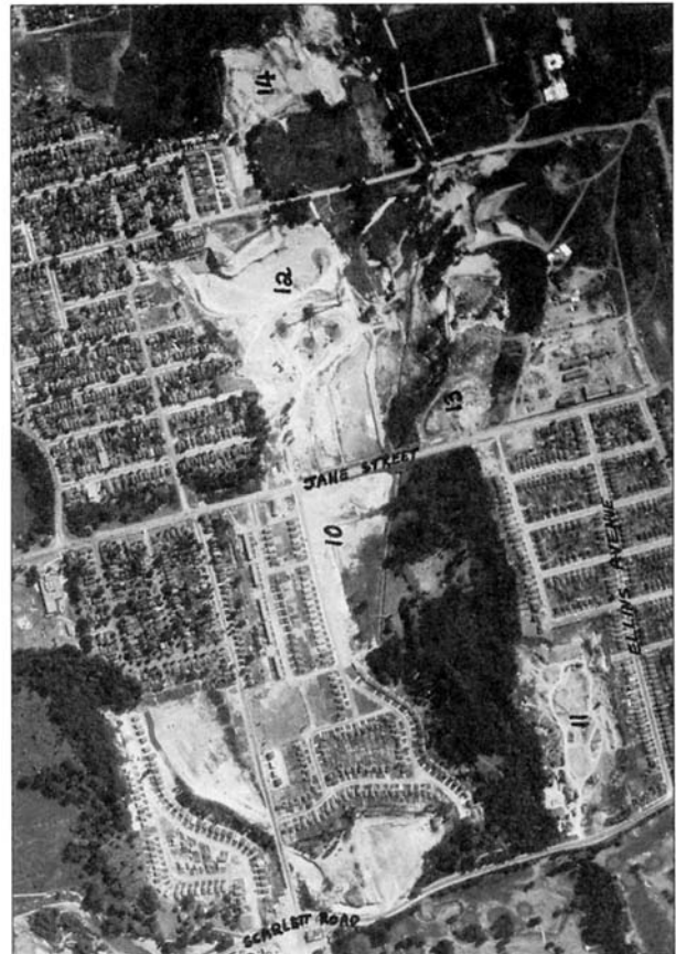
Photograph 7 In 1954, extraction activity at Jane Street - Alliance Avenue was still in full swing. Several sites which are now rehabilitated are identified on the aerial photograph.
