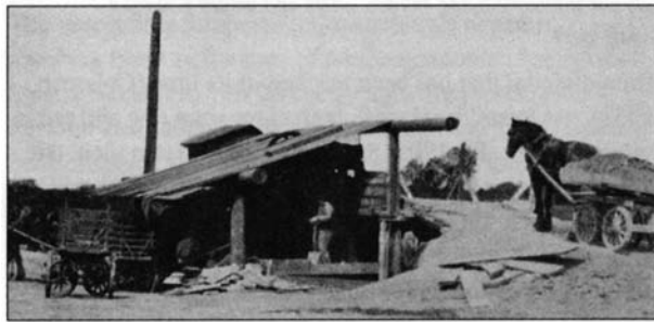
Photograph 4 Simple soft-mud plant at Chapman Brick Company, Dawes Road operating in 1930. In a five month season, the plant produced 2 million bricks.
