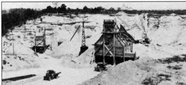
Photograph 6 Scarlett Plains sand pit, east of Lambton Golf Course is now part of a housing development. In 1932 it was a bustling and productive extraction site as motor vehicles began replacing the horse teams.
