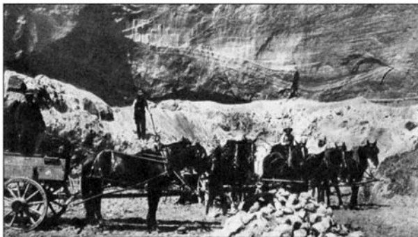
Photograph 11 Shaw Street sand pit was excavated in a 24 metre deposit of crossbedded, sandy materials. Willowvale Park now occupies this site.
