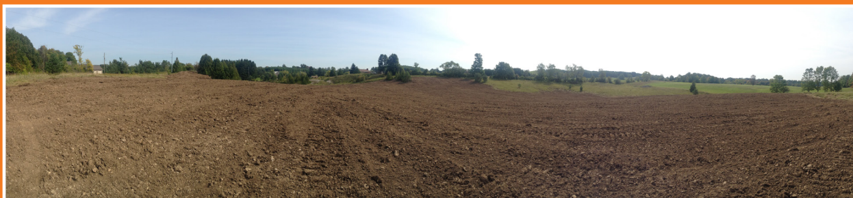
Figure 2b. During construction.
