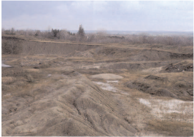
Figure 8. Abandoned pit. Severe erosion problems could have been controlled by regrading, soil amendments, and plantings.
