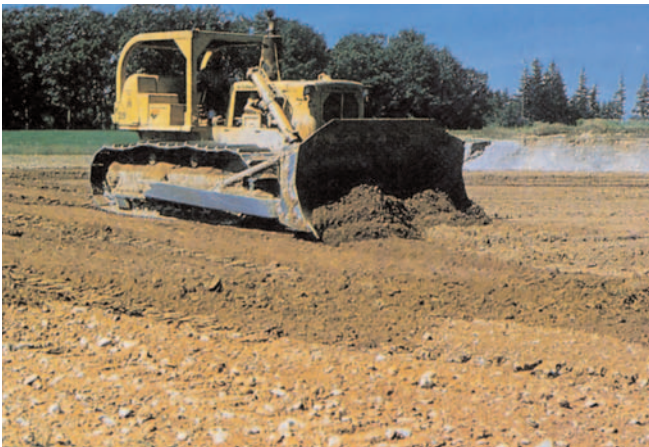
Figure 8. Topsoil is spread and levelled with a minimum amount of handling to reduce soil compaction.
