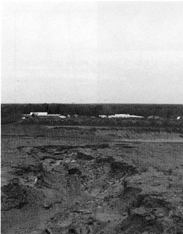
Figure 14. Costly soil erosion problems can result from inadequate soil stabilization and bare, steep slopes.
