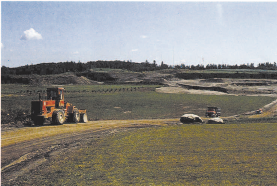
Figure 24. Pits can be rehabilitated progressively. The orchard in the centre of the photograph will be bearing fruit before extraction of the unused area is complete.
