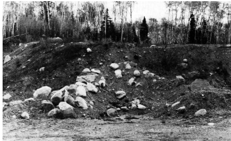
Figure 7. Very bouldery site cleaned, graded, levelled, and ready for seeding, Northern Region.
