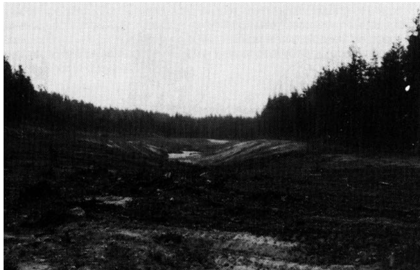
Figure 10. Ministry of Transportation and Communications site in Northwestern Ontario (same site as in Figure 2). Slopes have been graded and levelled, topsoil has been spread, and the site is ready for the application of seed, fertilizer, and mulch.
