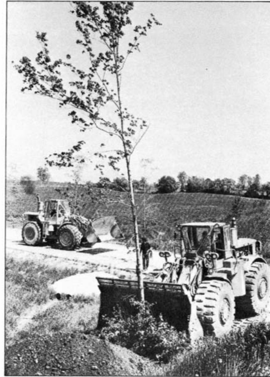
. . . and replant it in a new location (Note: greater success is likely with smaller trees and spring planting). (Custom Aggregates)
