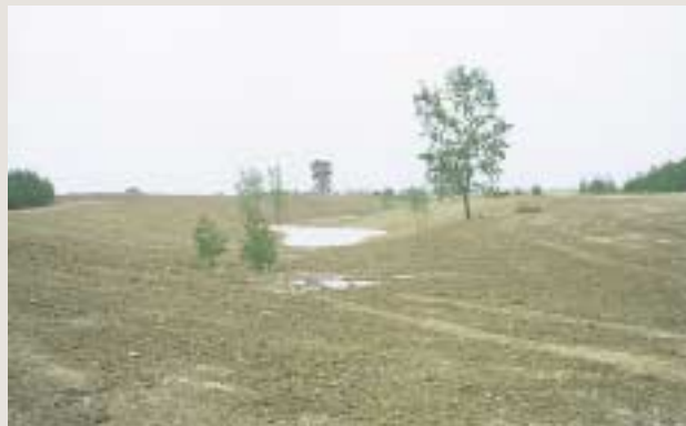
Following construction and prior to seed germination
