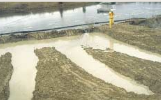
Wetland cell during excavation
