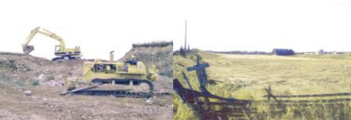
Podolski property - Before and after rehabilitation
