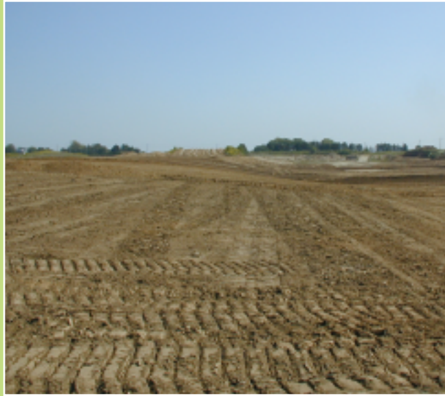
Rough grades (looking east)
