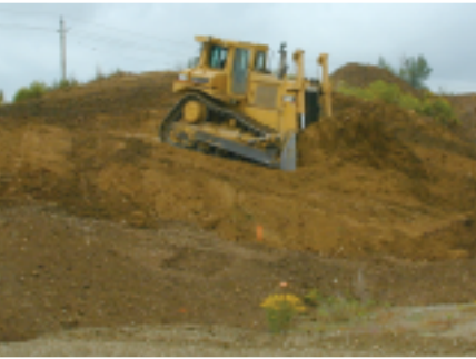
Dozer pushing soil from boundary berm
