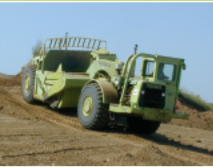
Motorized scraper moving soil for placement on pit floor
