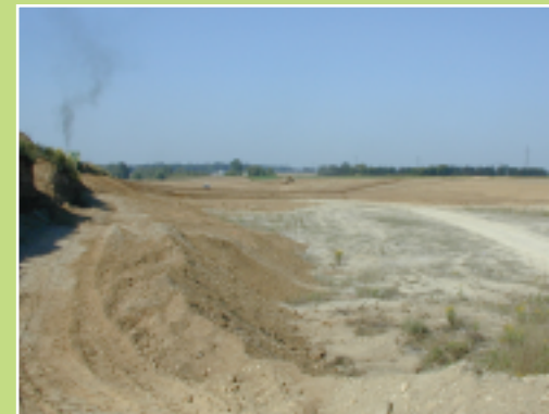
Site grading commences (looking west)
