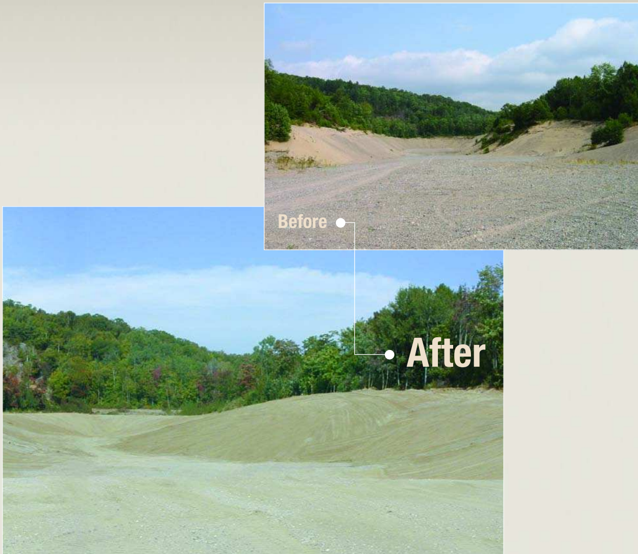
Grading completed – seeding has yet to germinate.
