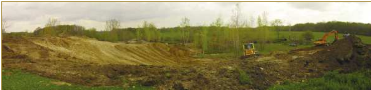
MAAP Rehabilitation in progress Spring 2005
