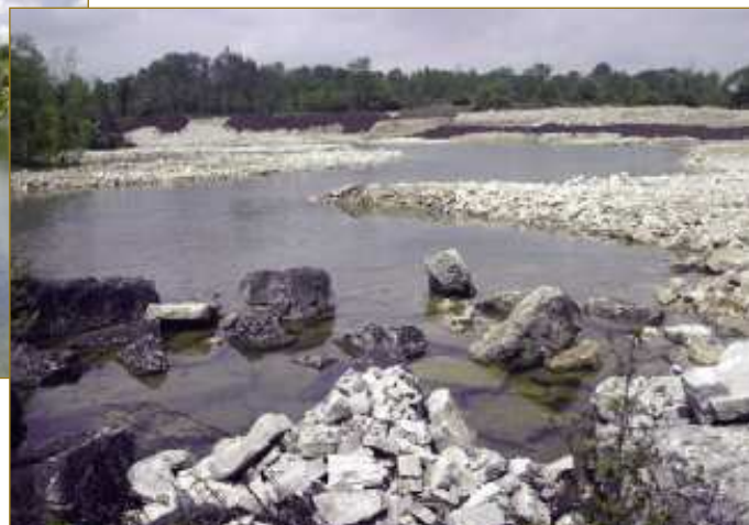
Fletcher Creek Quarry immediately following construction.
