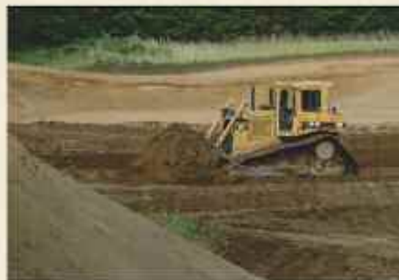
The abandoned sand pit has been leveled to minimize environmental variability in the research area.
