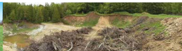
PROJECT #13-03A, BEFORE
