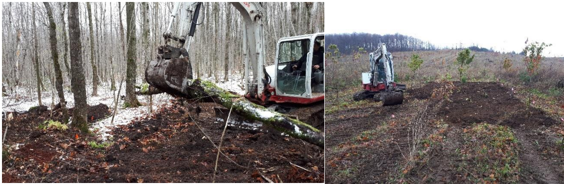
Figure 1: Example of operators extracting Living Mulch (LM) from a donor site then redistributing it at a recipient site
