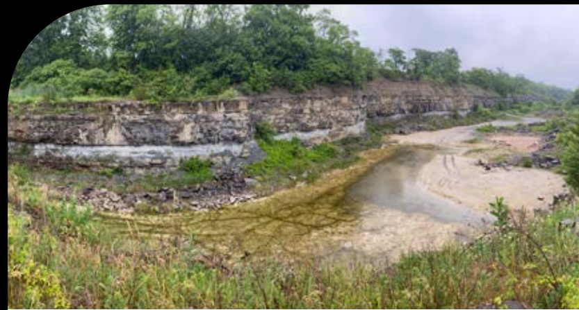
East section of quarry that requires site-safety improvement near the main driveway and relocation of fill material and debris.
